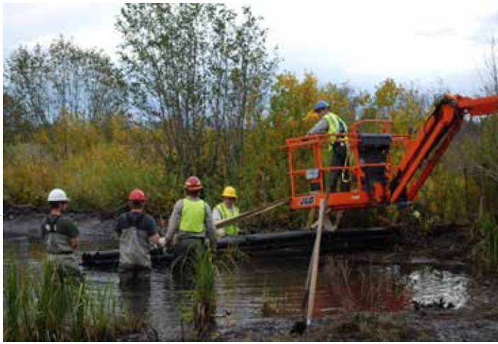
Maintenance workers helped resource staffers design and install a “beaver deceiver” in a pond so the animals would not be displaced.
