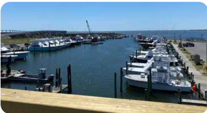
Oregon Inlet Fishing Center: Once nicknamed “the creek,” a former tidal creek turned into a water parking lot for fishing boats.
