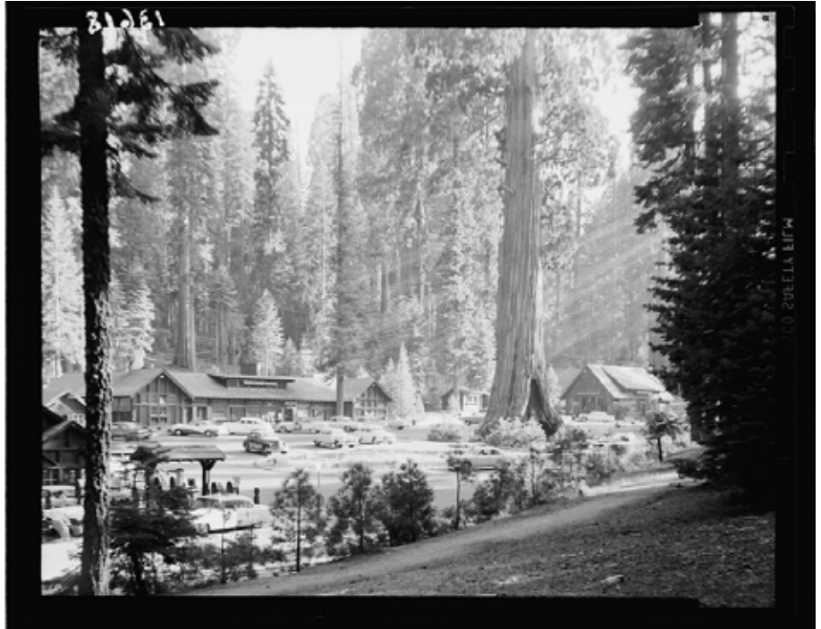
The Giant Forest Market gas station, market, and other developments as they appeared in around 1955. Photo credit Library of Congress
